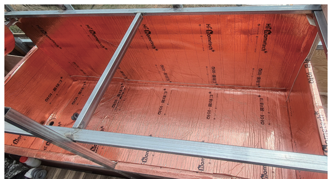
Inner part of the fish tank covered with foam board insulation
