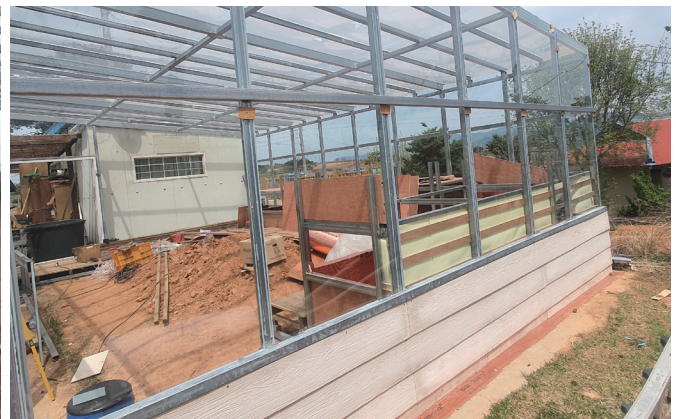
Gluing glass sheets and windows onto the steel frames
