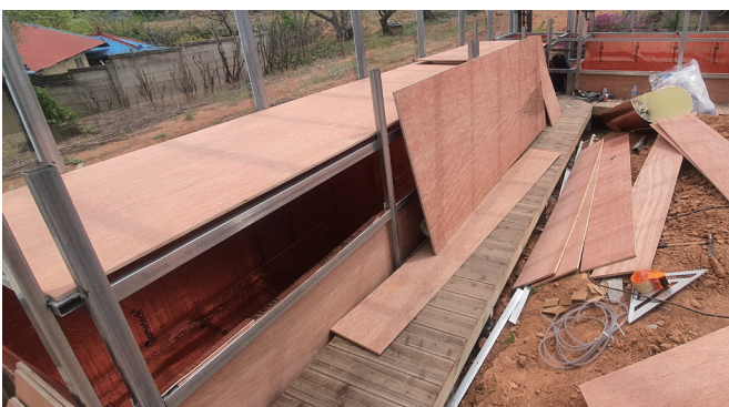
Installing fish tanks on the lower level
