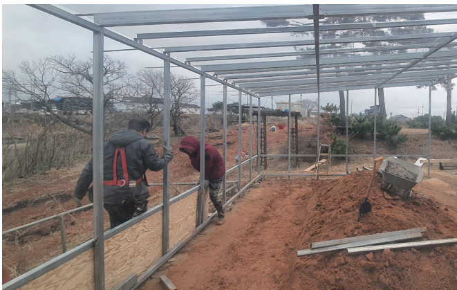
Nailing wooden panels and foam board insulation to the steel frames
