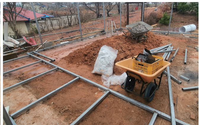
Leveling the ground and installing steel frame support for the deck
